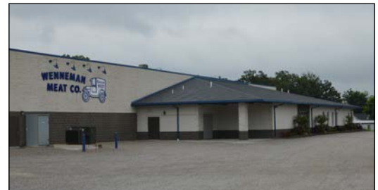
Wenneman's expanded processing facility and grocery store, completed in late 2011.
