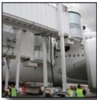
Passenger Boarding Bridges
